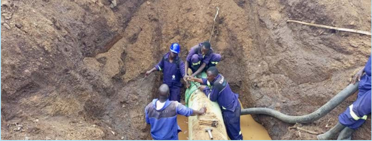
Non-Revenue water technicians installing a clamp on a water pipe.
