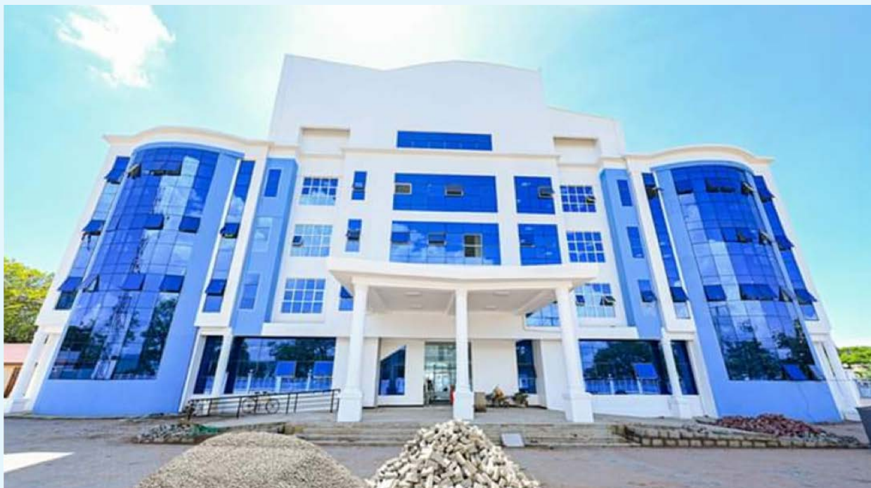
New office block ongoing construction
