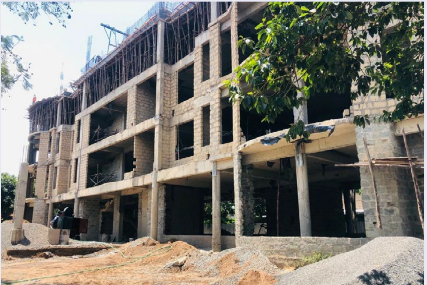
New office block construction in progress
