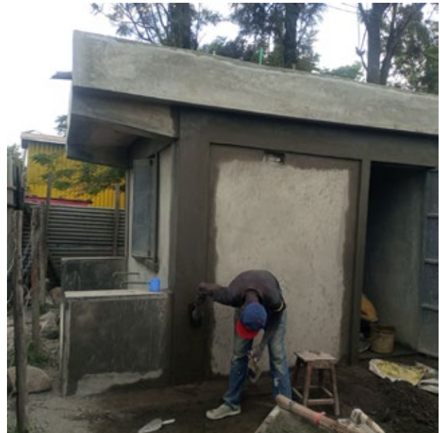
Water kiosk under construction
