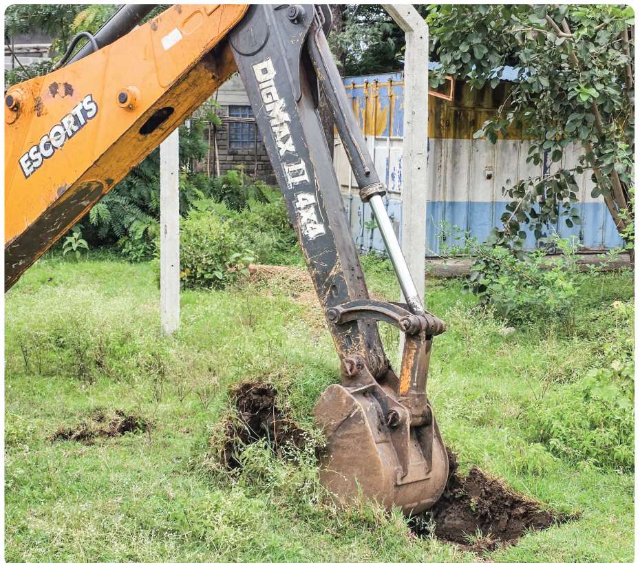
Photo file: Ground breaking
