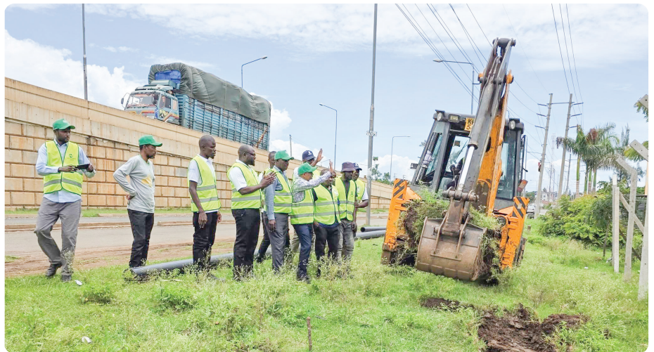
Photo file: During the project ground breaking at Kachok
